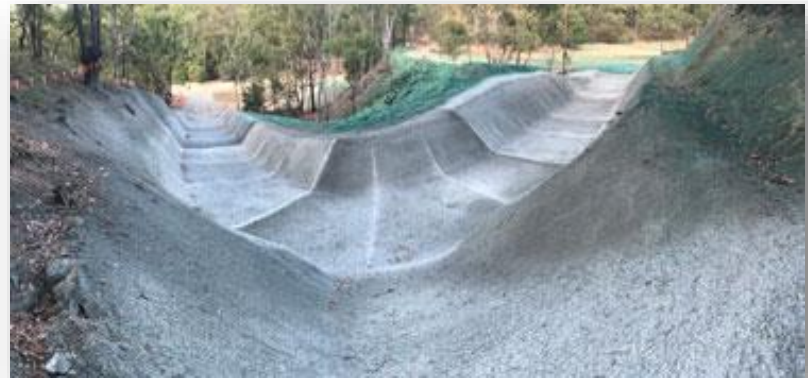
Target Gully tailings dam: redesigned spillway 1
