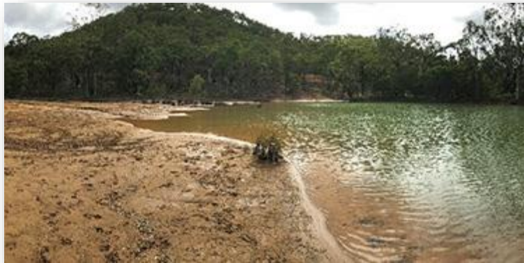
Target Gully tailings dam: before remediation work 1
