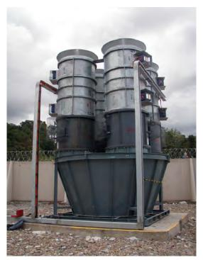
Figure 9 4 x 2 x 55 kW (110 kW) 1.250 mØ fans blowing into RB3 single 2.2 mØ intake raise on surface
