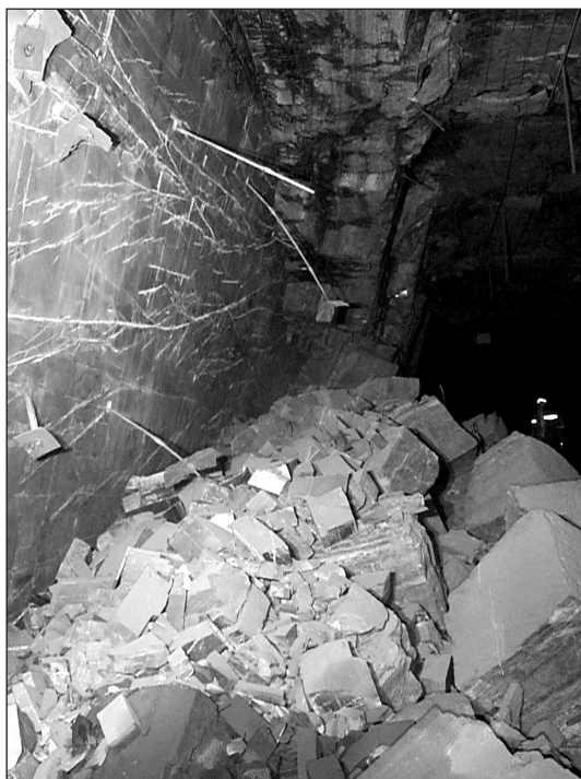
FIG. 2 An example of rockmass deterioration (in the hangingwall of sill drive) induced due to stress changes, a small-sized pillar and production firings from an adjacent bench (photograph looking north). Despite the level of damage, the associated rock noise was found to dissipate relatively quickly
