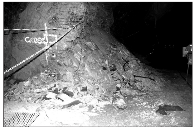
FIG. 13 Photograph looking south of 14CBLH, 19/19A Sublevel, showing the shallow dip of the orebody
