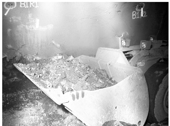
Figure 7. Typical size of the failure material from J46 fault exposed on P3849 SEDR, 20B (note that the unit mucking from the failure zone is an Elphinstone R1700).
