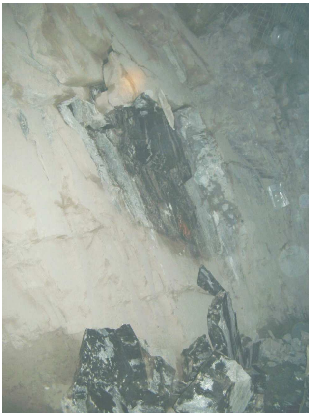
FIG 6 - Time dependant loosening of wallrock in the Main Lode Decline.
