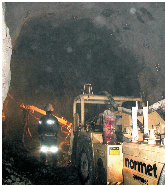
FIG 7 - Hydro scaling in progress.
