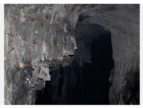
Before: This photograph shows obvious overbreak with damage to screen and bolts owing to a pattern that was too tight (blastholes too close together).
